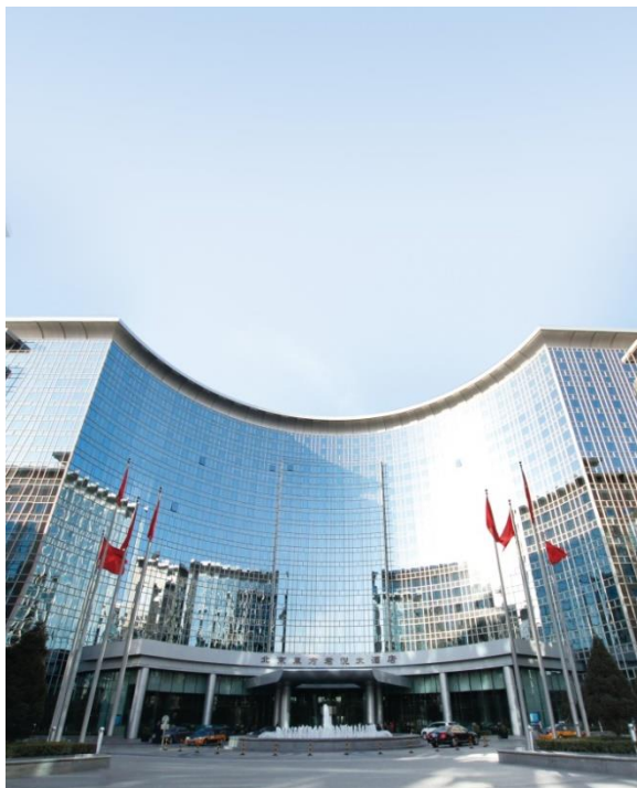
(2) As an integral part of Beijing Oriental Plaza mixed-use development, Grand Hyatt Beijing is one of the leading five-star hotels in Beijing featuring 718 guest rooms and suites.
